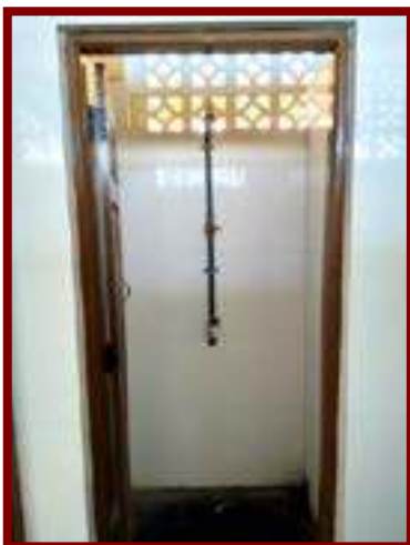
Improvement of Rest rooms Keerimalee ,Jaffna
